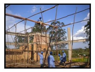
Once all the cut steel has been welded into place, each roof support is carried along the top of the scaffolding and then carefully lifted into place. It takes eight men to carry and manoeuvre each of these heavy sections and there is only a small margin for error. Each section fits on to a notched out part of the reinforced concrete top of the walls. These many marked out portions were achieved using a lump hammer and chisel.
